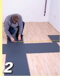
Measure the length and width of the room and divide the demensions in two. Locate and mark the centre of the room. This is the approximate starting point for the installation. Check the number of full tiles and the width of part tiles required to reach the walls in each direction.
