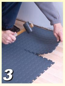
The files are designed to fit tightly together. Use a rubber mallet to hammer the tiles into position. On reaching the walls, cut the edge tiles so as to leave 1/4in wide gap between tiles and the wall.
