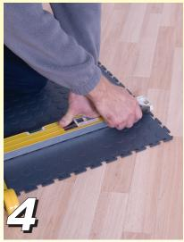
Cutting the edge tiles should be done with a sharpe blade. A good non-slip straightedge should be used. It is better to make several light cuts than one heavy cut. Always cut the tile from the front. A cutting board should be used to prevent damage.
